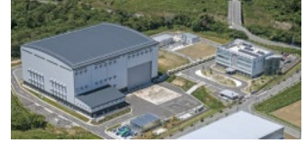
Naraha Remote Technology Development Center
