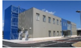
Collaborative Laboratories for Advanced Decommissioning Science
